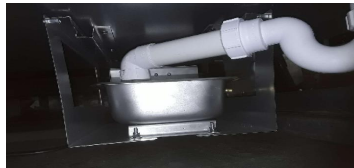
Picture 2; Drain outlet position
